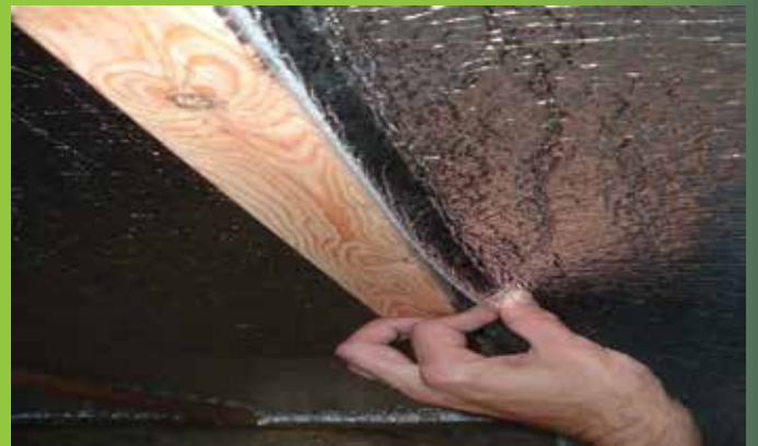
.....Staple To Inside Corner Of Joist
