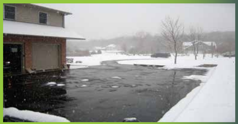
Snow Melt System After
