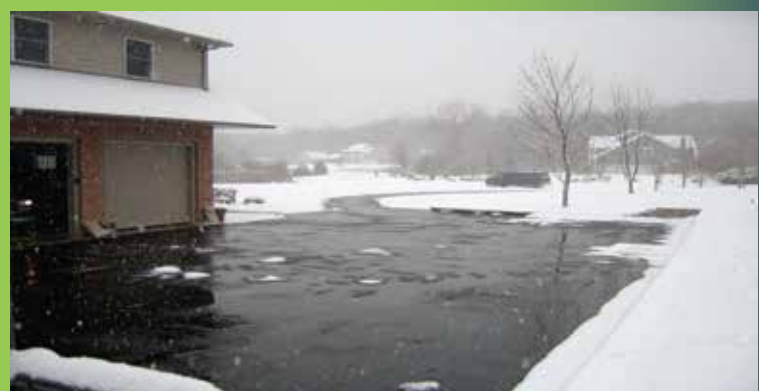
Snow Melt System After
