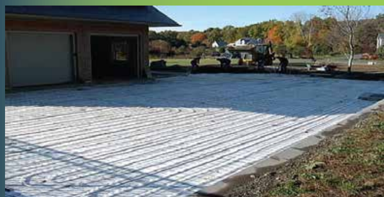
Snow Melt System Before
