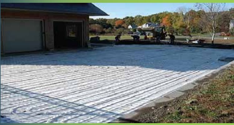
Snow Melt System Before
