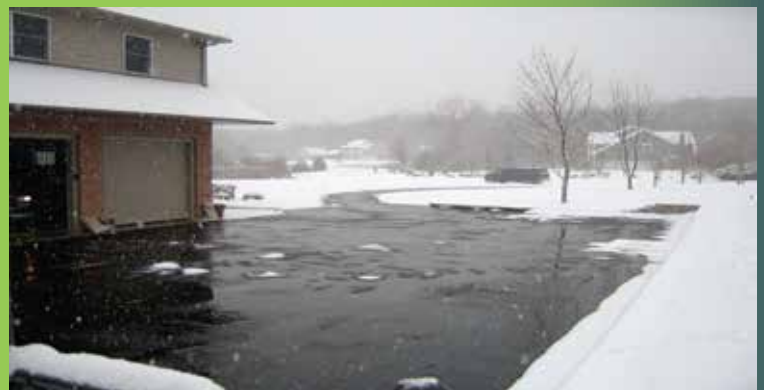
Snow Melt System After
