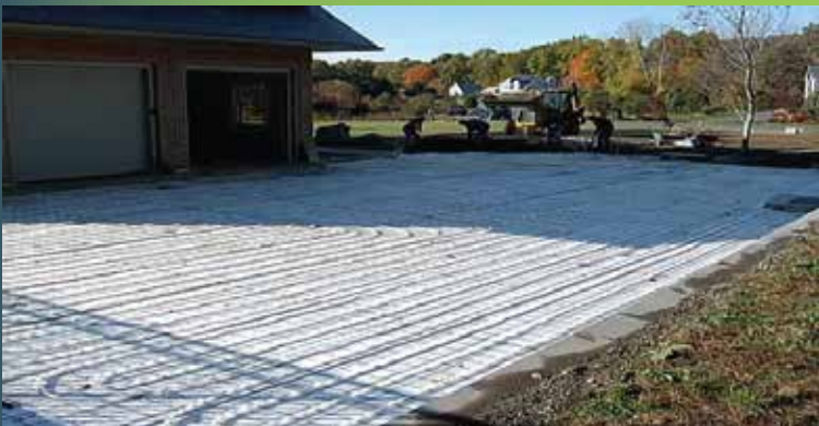
Snow Melt System Before
